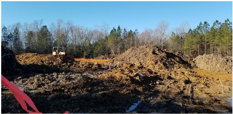
Earth Moving—Site Work
